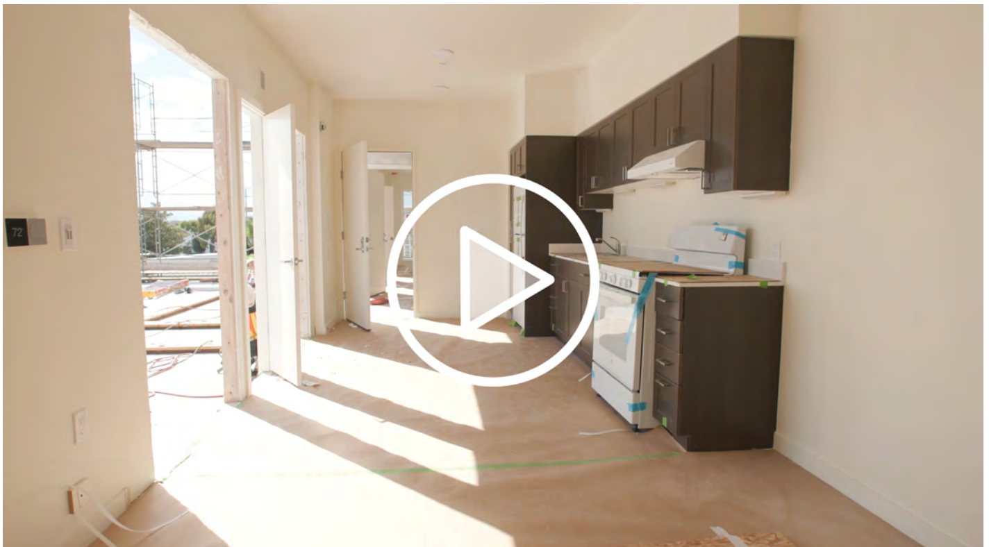
Assembled onsite and up to 80% complete in weeks, the building needs quick protection from rain.
