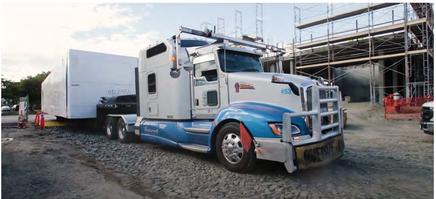
Completed modules are shipped from factory to a 'laydown yard' near the final site.
