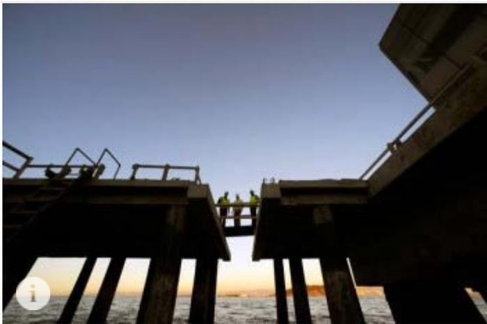
museum and protect it from earthquakes. The need to refurbish and seismically upgrade the piers meant construction would take place not only above the San Francisco Bay, but also below it, where piles extend more than 160 feet into the bottom of the bay.
