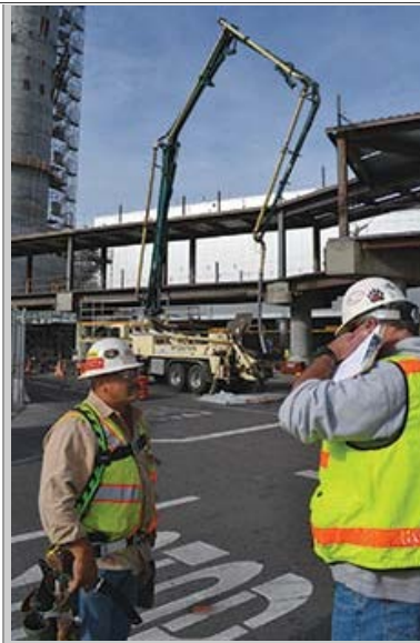
Carpenter foreman Tommy Molina, Local 405, and Superintendent Rich Gile, Local 713, at SFO control tower site..
