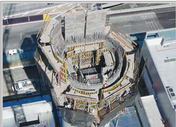
Aerial view of new SFO control tower as construction nears completion.
